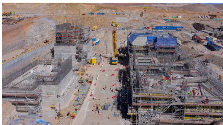
Construction of Quebrada Blanca Phase 2. Credit: Teck Resources
